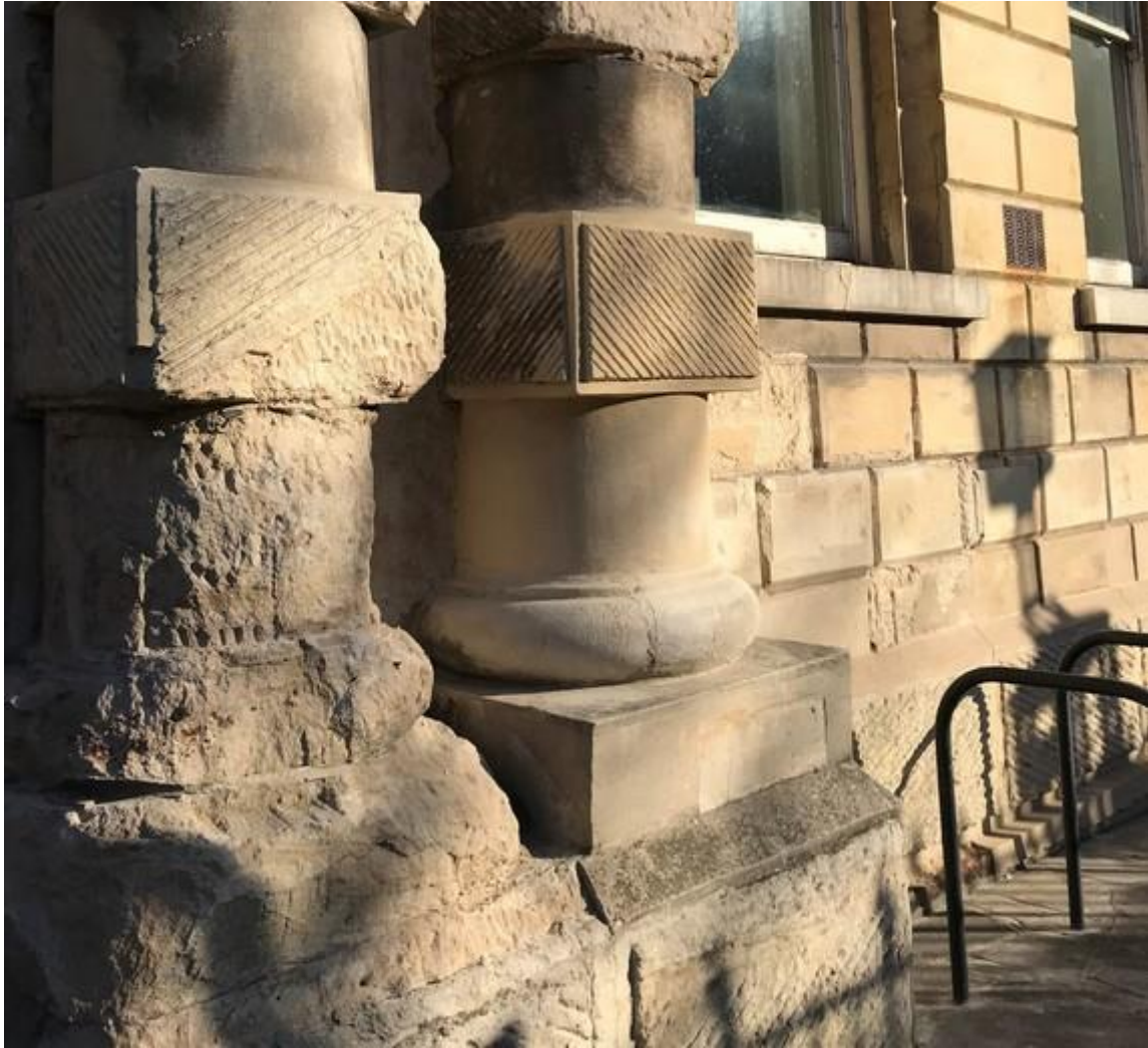
Before and after! The left-hand column has yet not been restored while the lower section of the one on the right was completed last week as a demonstration.
