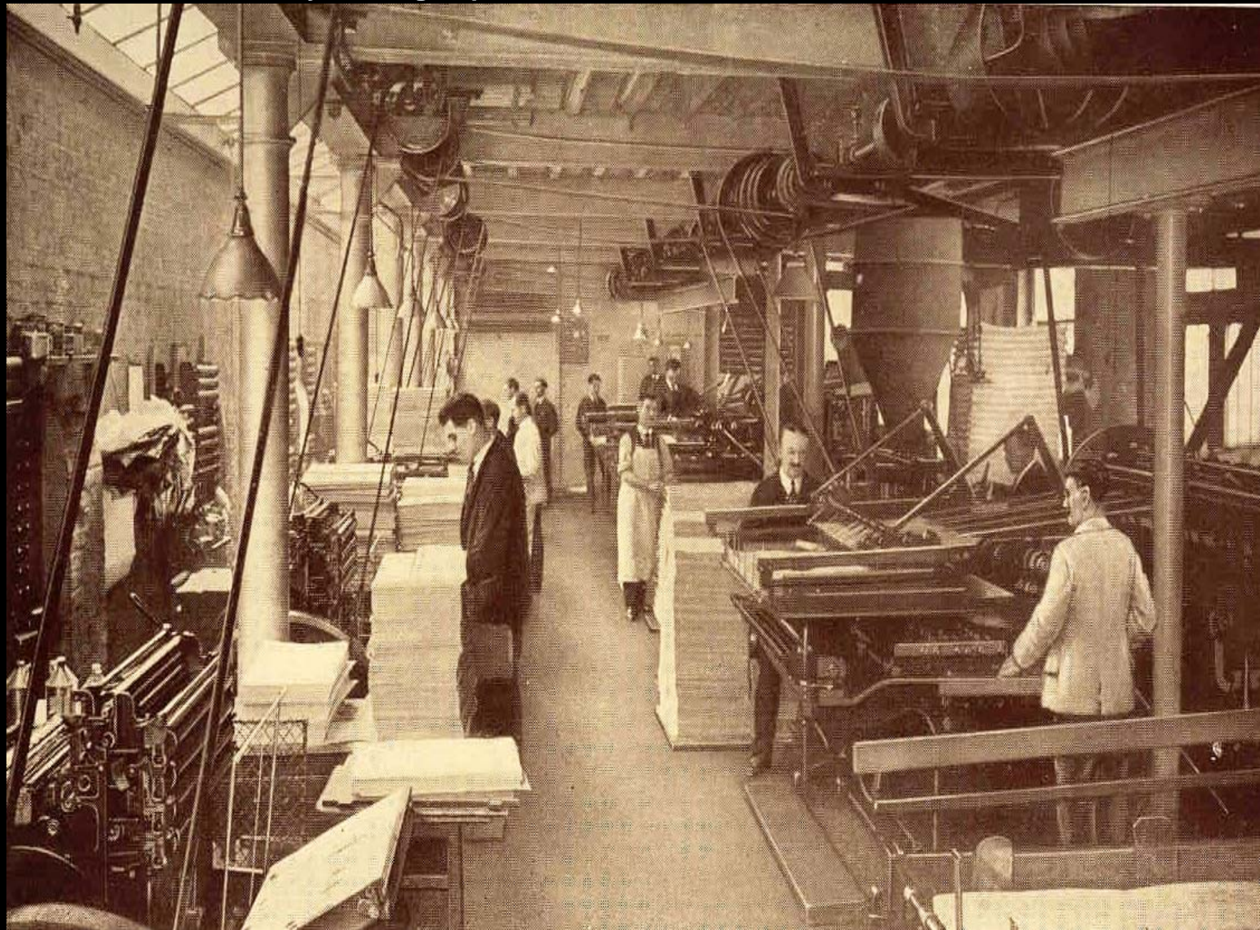
Work: Allen and Hanbury Printing Department, one of the machine rooms, 1927
