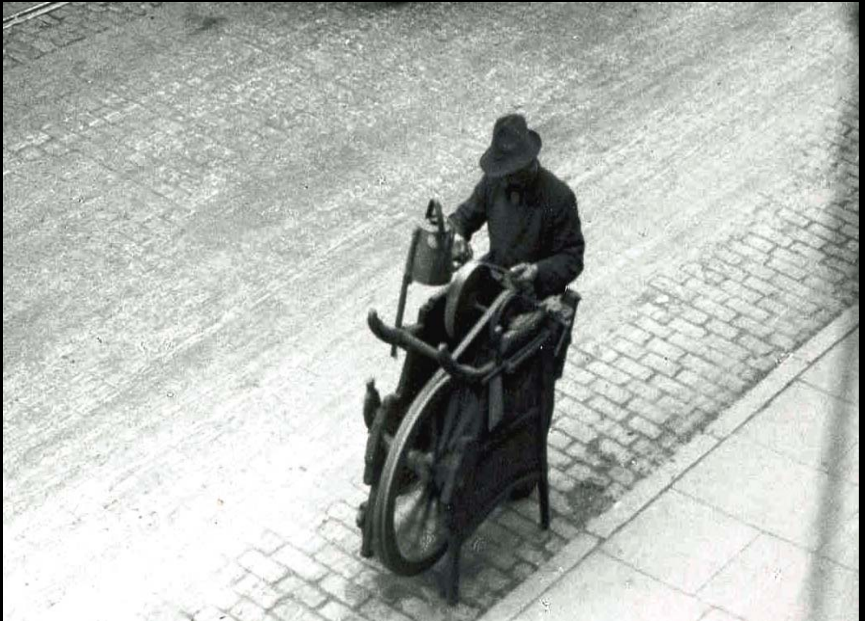
Work: Knife grinder, East India Dock Road, c.1930
