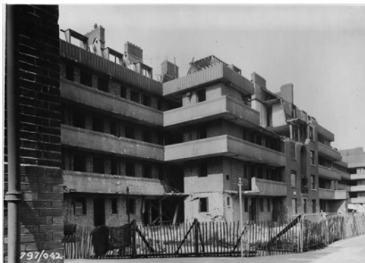
Ring House, badly damaged
