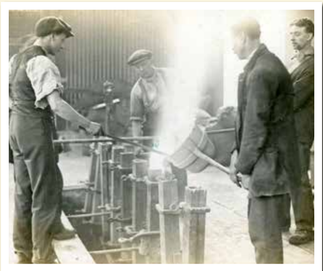
Casting gun cases at the Commercial Gas Company Munitions Foundry, Stepney, c 1916.
